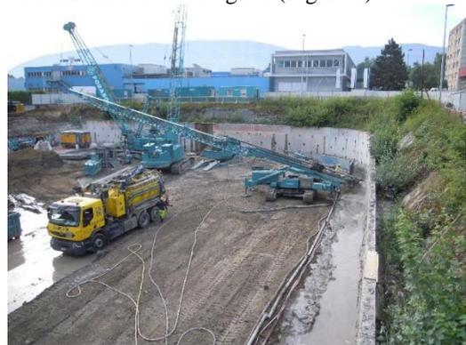
**Figure 6:** effective spoil management (storage bund and pump truck)
