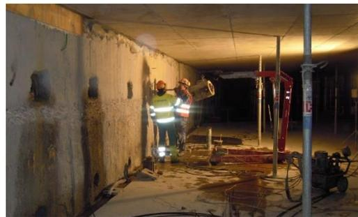
**Figure 8:** anchor free length extraction
