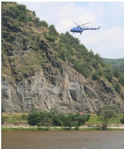
**Figure 8.** Rockfall protection and rockfall mitigation on railway section Všetaty – Děčín, Czech Republic.
