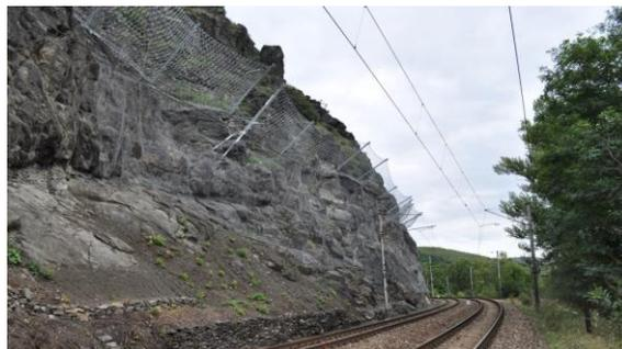
**Figure 9.** Rockfall protection and rockfall mitigation on railway section Všetaty – Děčín, Czech Republic.
