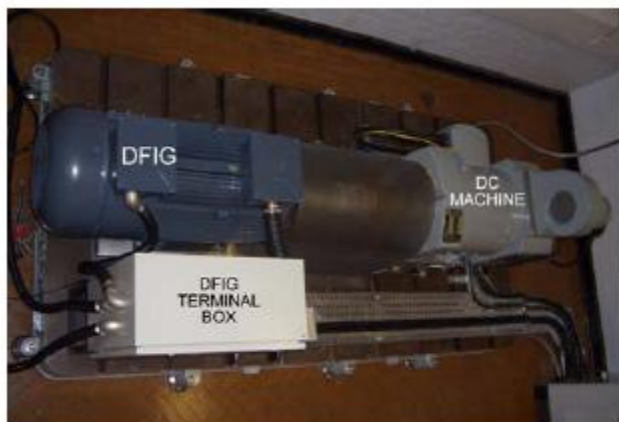
Electrical Generator Test Rig
